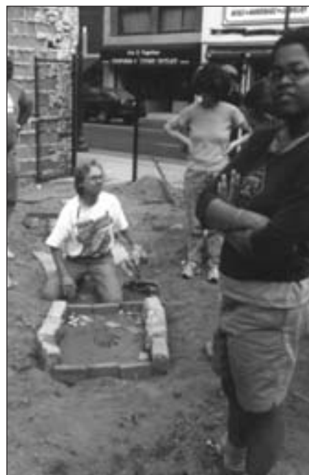
Ron Oster, a volunteer with the Park on Nash group, demonstrates how to build a concrete path.
