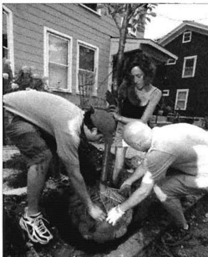
Placing a Tree into a Newly Opened Tree Pit
