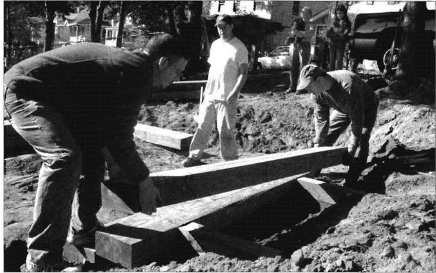
Mark and David Lift the Heavy Wooden Steps in Place
